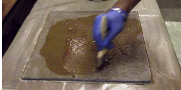
4.2 (c) Repair surface preparation
